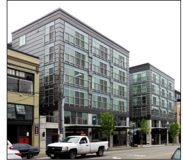
The modulation or division of this building into two sections with a recessed middle portion helps to keep it in scale with the neighborhood.
