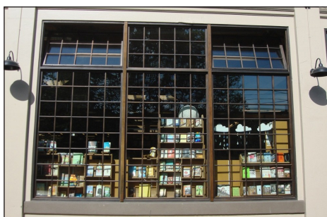
Window trim detailing.
